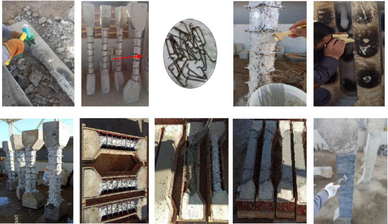
Fig. (6). Sequential steps of RC column repair.
