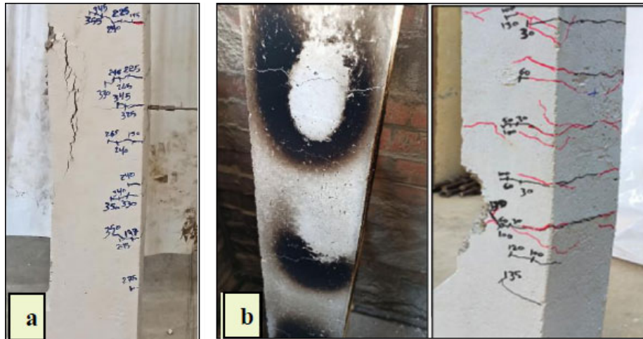
Fig. (15). Spread of crack in specimens, a. Column specimens without fire, and b. Column specimens with fire exposure.
